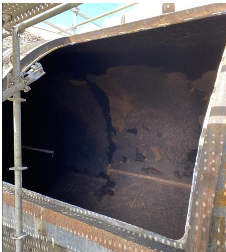
Figure 11: Cut-out for Temporary Access Point 3
