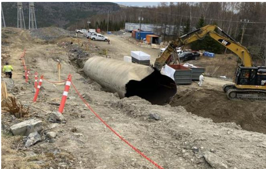
Figure 6: Excavation and Demolition Cans 2 to 8
