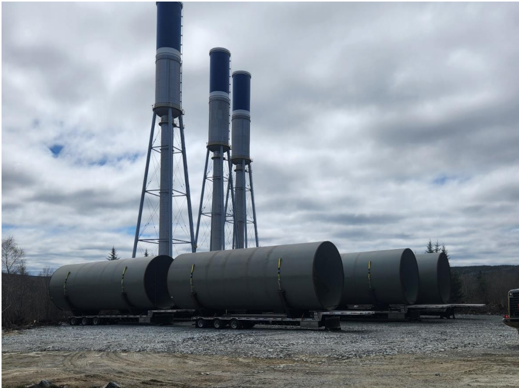
Figure 5: Staging of Penstock Sections in Marshalling Yard
