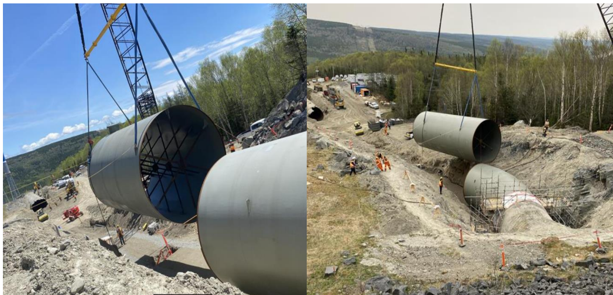
Figure 10: Placement of Cans 3 and 4
